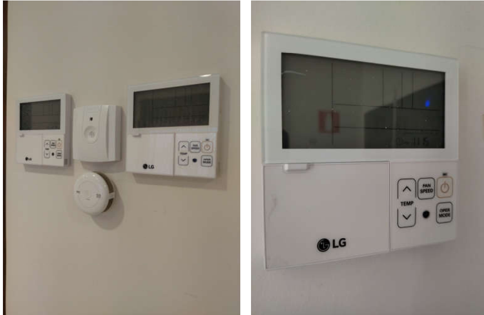
Figure 8. Thermostats installed in KRIPI building.
