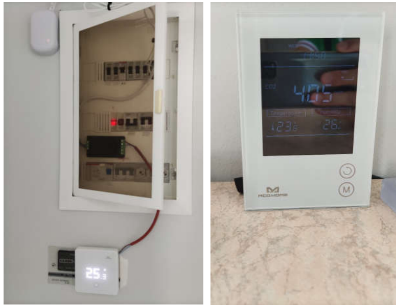
Figure 86. left) Clamp meter and boiler thermostat, right) Temperature, Humidity and CO2 sensor.
