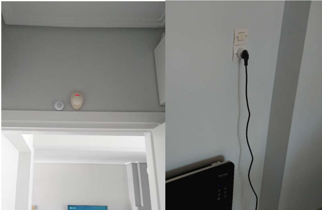
Figure 83. left) Motion sensor installed in the corridor, right) smart plug installed on the convector.
