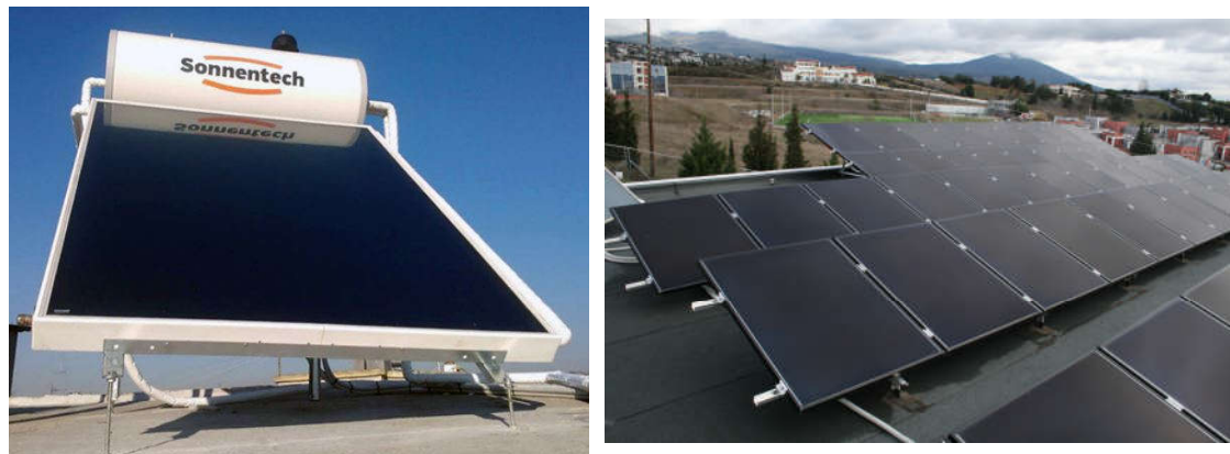
Figure 10. left) The solar water heater, right) The photovoltaics installed on the roof of KRIPIS building.
