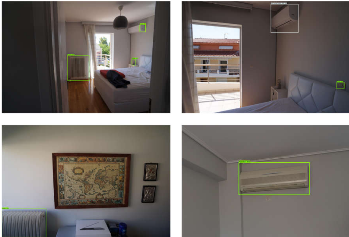
Figure 94. MEP objects identified in the CONKAT apartment
