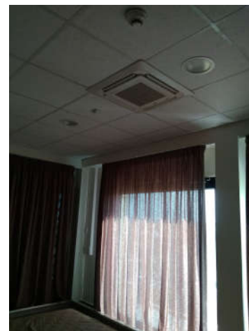
Figure 7. left) The outdoor units placed in KRIPIS building, right) 4-Way Cassette indoor unit placed in KRIPIS building.
