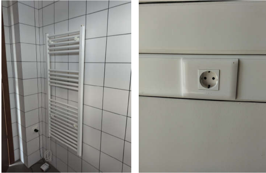
Figure 9. left) The electric radiator, right) the outlet installed in KRIPIS building.
